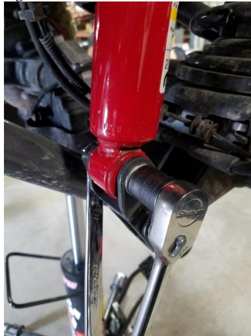
Figure 5. Bolting Shock to Extension Installation is Complete
